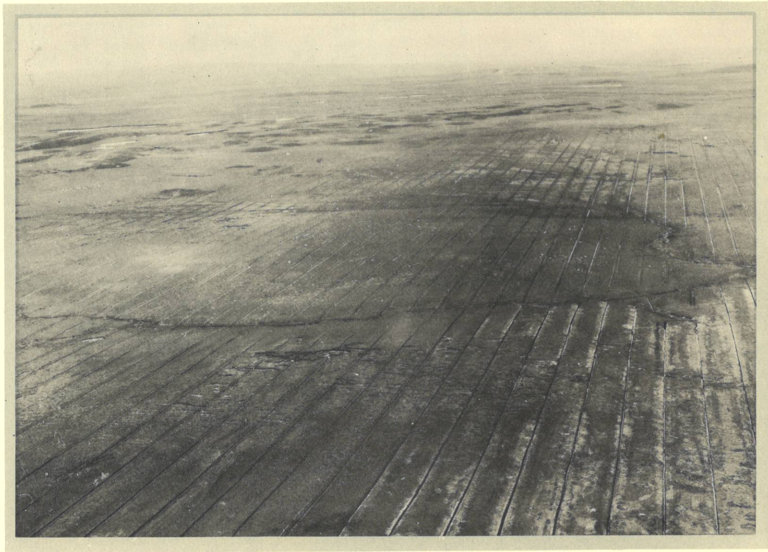
MILLED PEAT BOG BEING DRAINED INITIAL PLOUGH AND DISC DITCHER DRAINS SPACED AT FIFTY FEET INTERVALS
